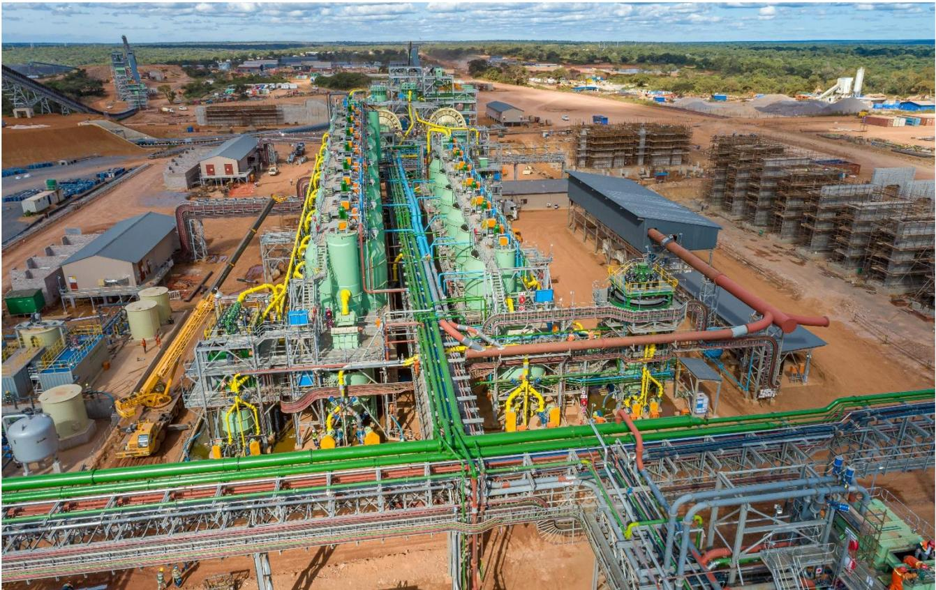
**Structural steel erection, platework installation and piping and valve installation for the first concentrator plant is effectively complete, as is electrical, controls and instrumentation installation.**
